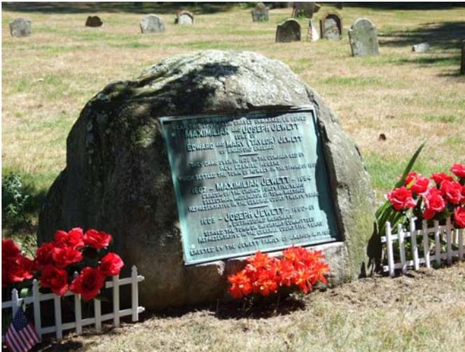
Akepox 2030 Epoxy. All sunken and or leaning stones will be reset with a washed sand and pea-stone gravel mixture to the proper height. Some of the slate gravestones are de-laminating at the top. These open cracked stones will be in-filled with a non-portland cement, color matching mortar, Jahn's Restoration Mortar. The Bronze Plaques will be lightly cleaned, buffed, and waxed to protect them.
